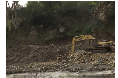
San Ysidro Creek Debris Basin in Santa Barbara County ( KEYT News )
